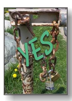
Note how proper gate locking has the lock on the end of the chains and through the State's lock (the master lock) as if it were the last link in the chain. The pin (not the lock) is put through the latch to hold it closed.
